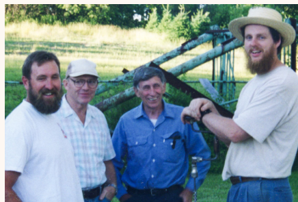
Pete Menard (3rd from left) with Ray Kerns, Richard Wells, and Jack Sobon, building the timber-frame shed in front of the historical museum, 1997.
