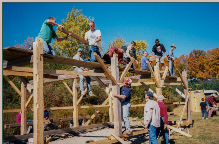
▲ In 1997, volunteers from the Historical Commission were joined by others in town to raise the timber-frame shed outside the museum. The shed was designed by Windsor's own master timber-framer (and Commission member), Jack Sobon.
