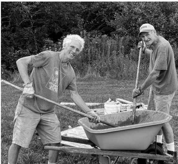
Tim Crane and Lenny Price preparing to install the new FOW chess/checkers table at Windsor Town Park.
